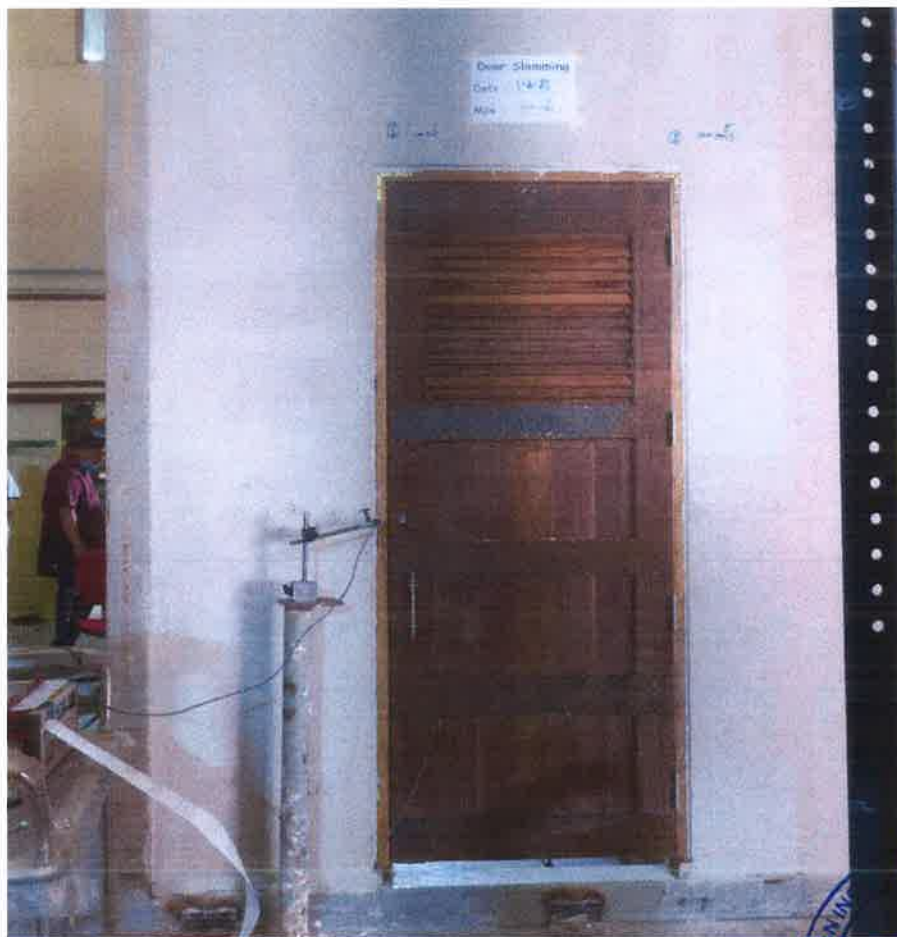
Figure 12 No partition damage after door slamming test
