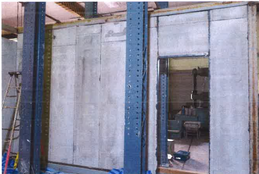
Figure 2.1 Wall during construction
